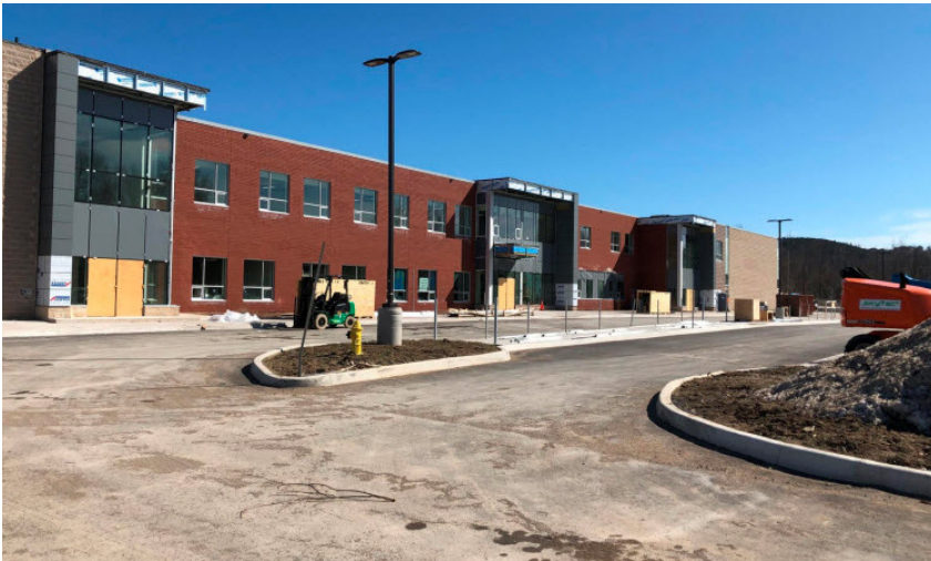
Georgian Bay Community School build project
